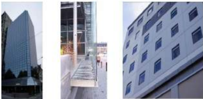
Fig. 4 : Light-medium weight cladding (left), Double skin facades (centre), and heavy cladding (right) [3]
