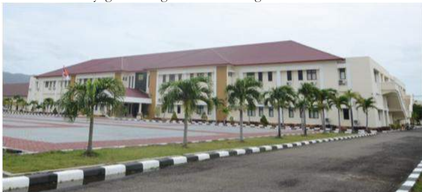
Fig.13 : The Prosecutor Aceh Office buildings from the out side
