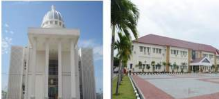
Fig.2 : A little amount of glass materials being applied in the latest office building in Aceh, Syari'ah court Aceh (left), Prosecutor Aceh offices (right)
